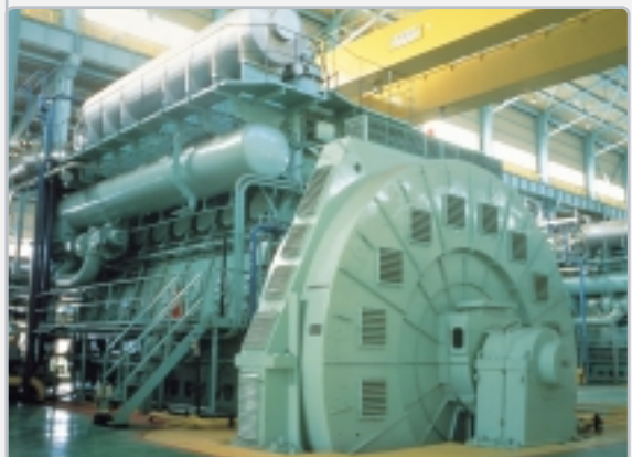
12,500KVA, 6.6kV, 52P, IP23
